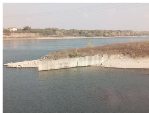
Figure 4.3 - Upstream spike of the embankment on the river side of the downstream berthing area at HPNS "Djerdap 2"
